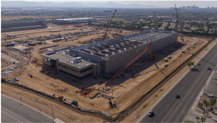
The QTS data center under construction in Phoenix Source: Wirestock Creators/Shutterstock
